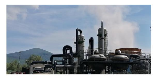
**Residues: adsorbent and filtering materials** are employed in AMIS to trap mercury and hydrogen sulphide from gas
