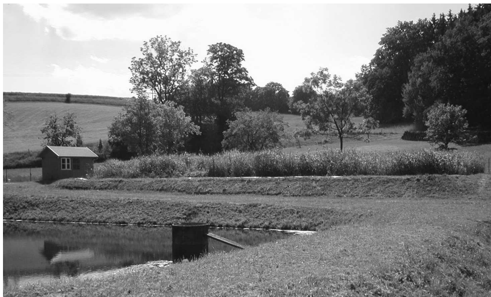
Fig. 1 Constructed wetland with a vertical and horizontal flow reed bed at demonstration site Wiedersberg, Saxonia
